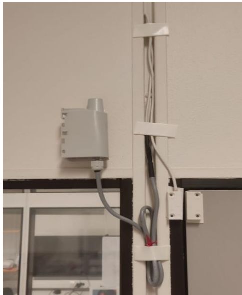
Figure 18: Contact sensor installed on the project room.
